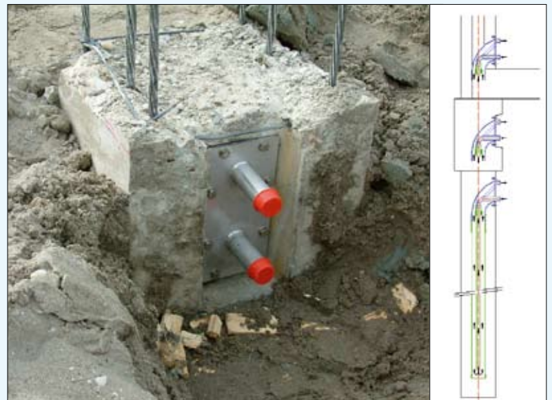
Another option is to use special piles doubling as heat exchangers. The heat extracted from the earth is fed through a closed circuit inside the pile to the heat pump.
